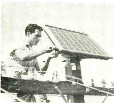
Rural telephone line now carries several circuits using transistor amplifiers powered by solar generator atop pole
